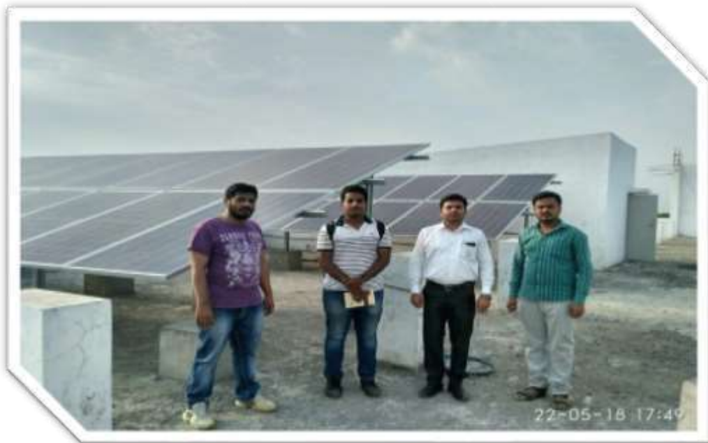
10 KW Jain Solar Panel
